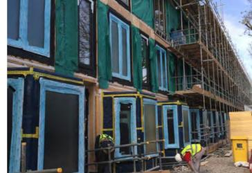
CLT components being assembled on site
